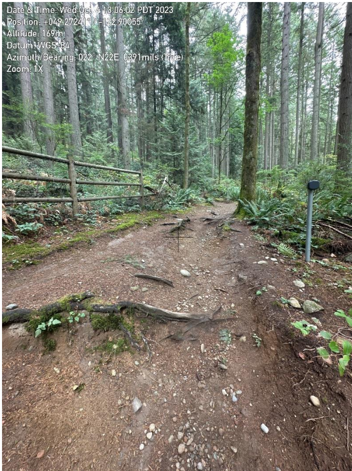
Photo 9: Severe erosion on trail. Trail widening visible on bottom right hand corner.
