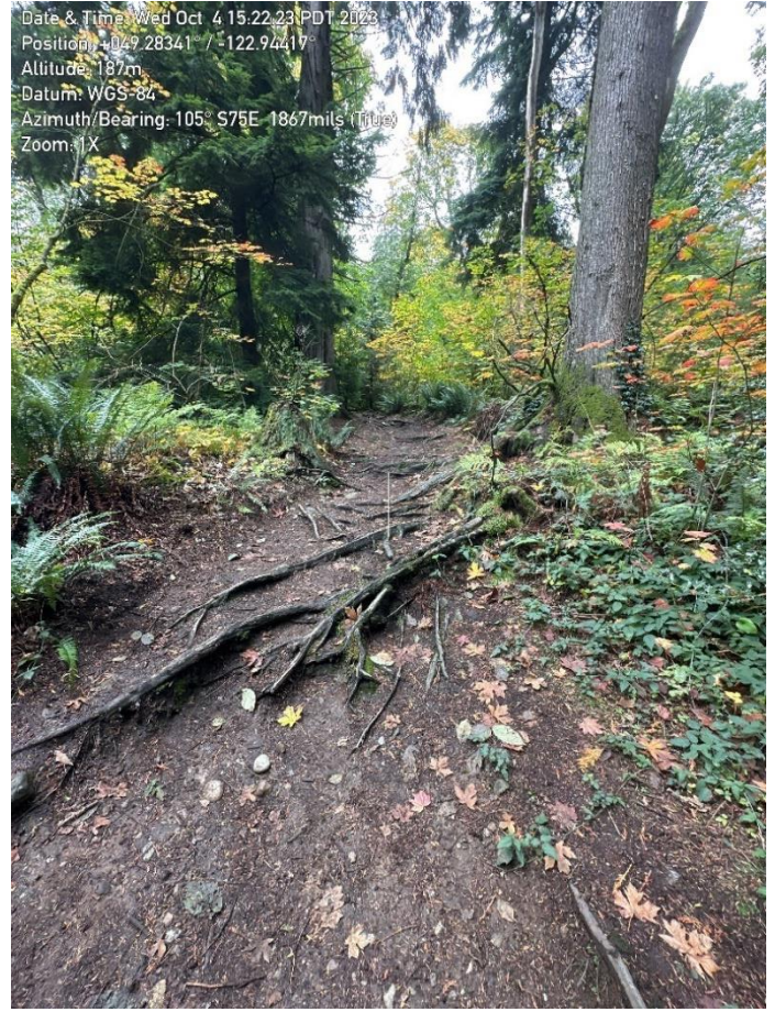
Photo 3: Severe erosion around tree roots
