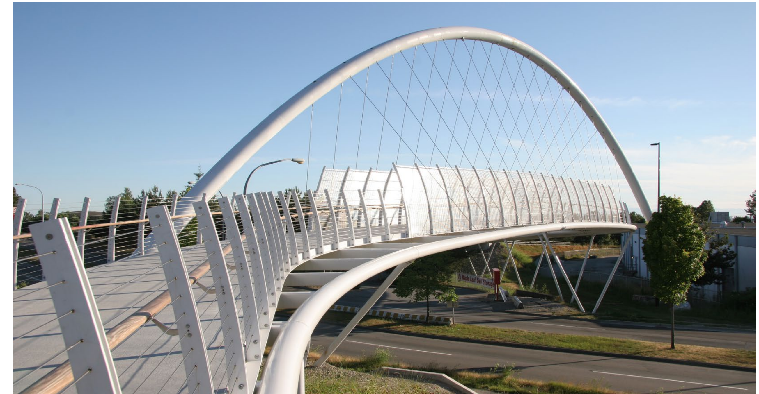
Overpass example near Griffiths Drive & 14th Avenue, Burnaby
